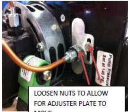
LOOSEN NUTS TO ALLOW FOR ADJUSTER PLATE TO MOVE
